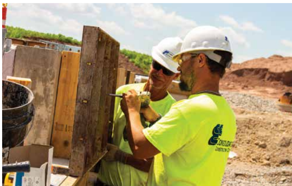
Photo provided by Consolidated Construction
